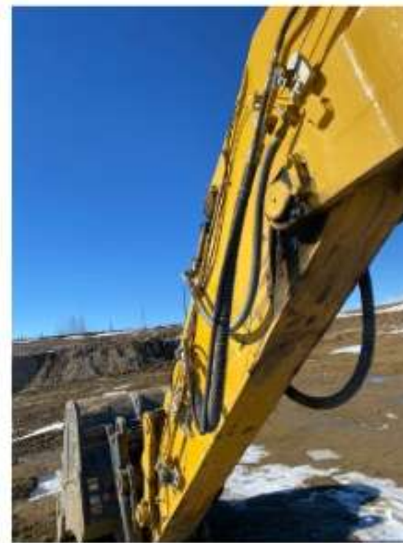
Hydraulic Leaks Photos
